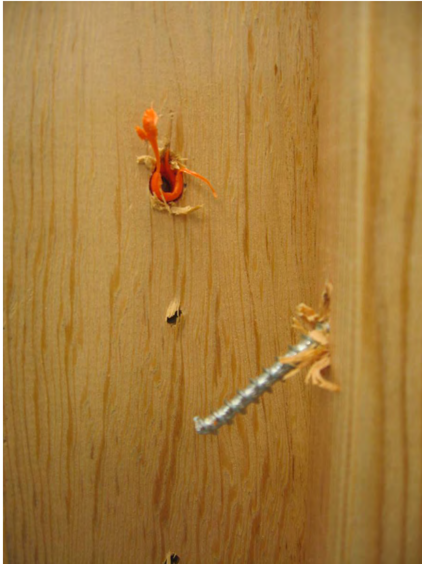
Photo No. 7 Deflector SP Fastener Pull-Out - Failure Detail
